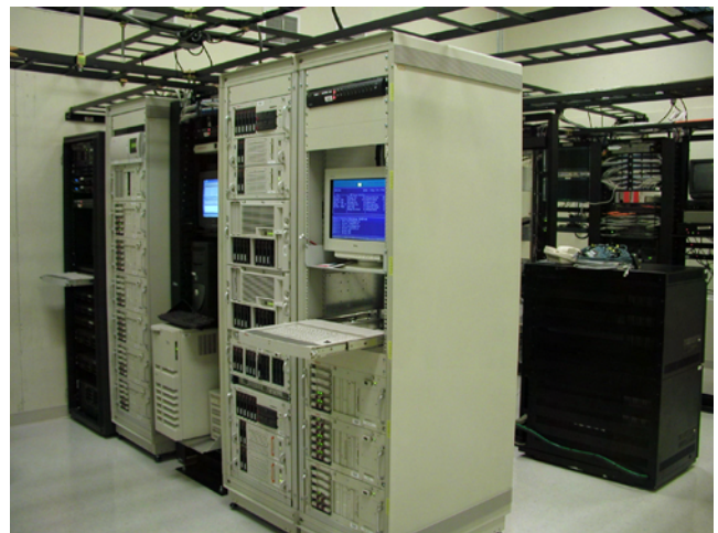
District Server Room
